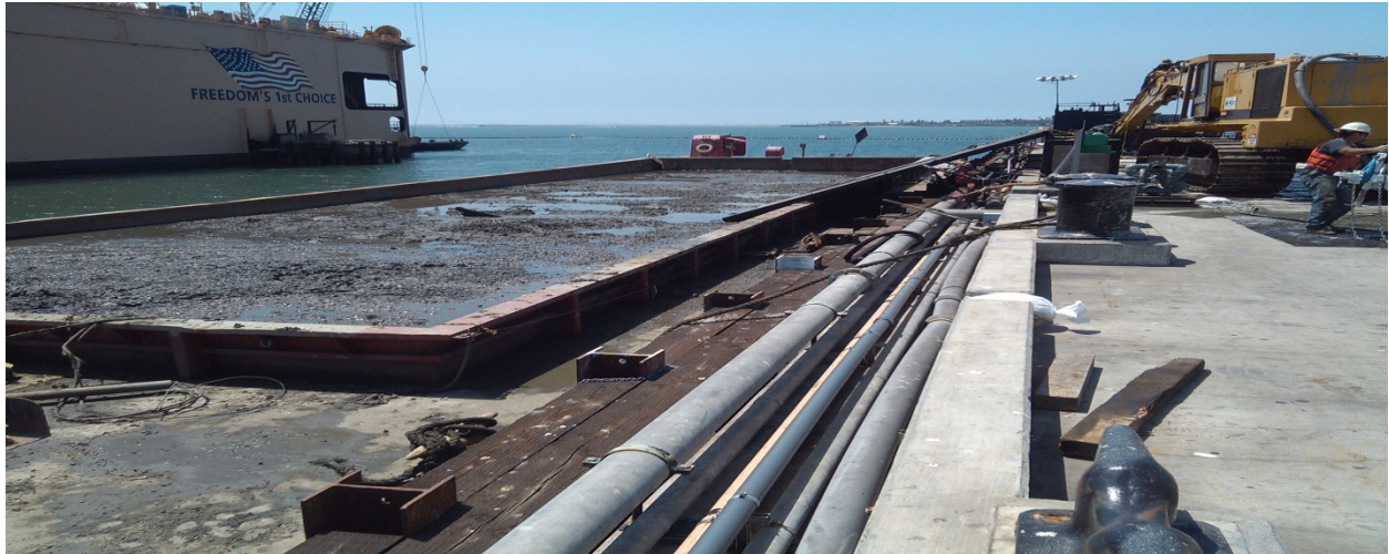
Sediment cement mixing in barge.
